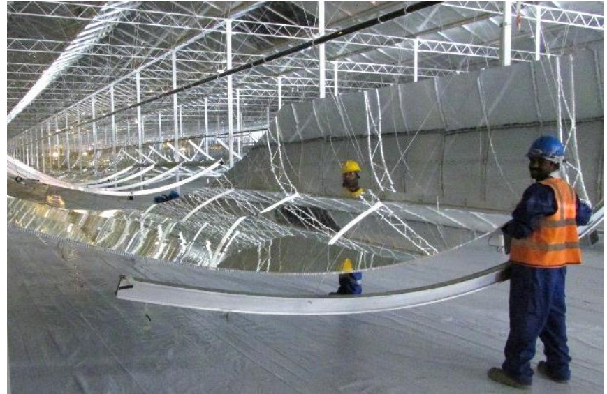
Interior tracking troughs GlassPoint Solar
